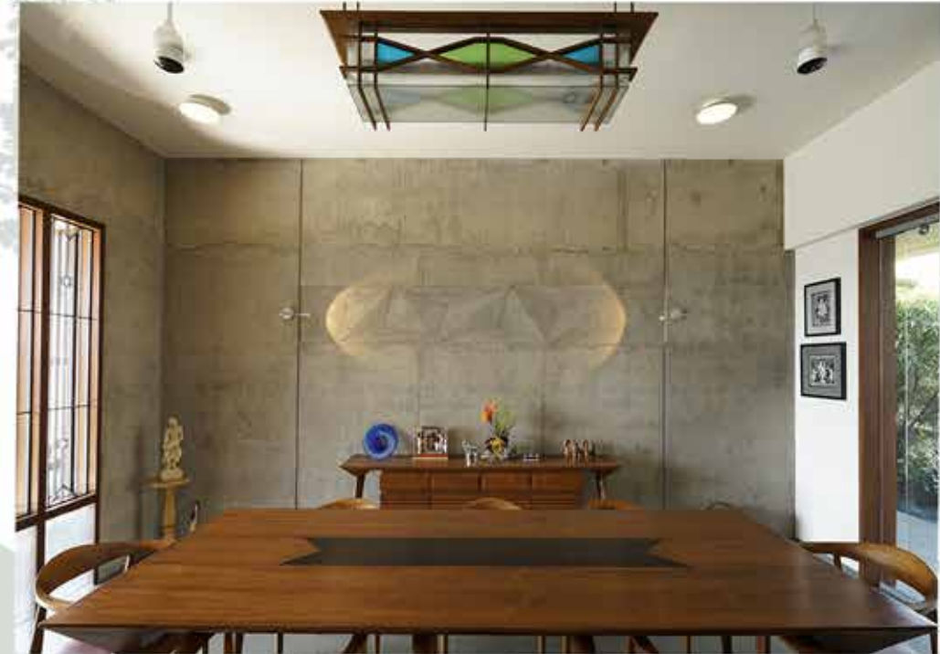
Exposed dining wall with pattern done with double shuttering
