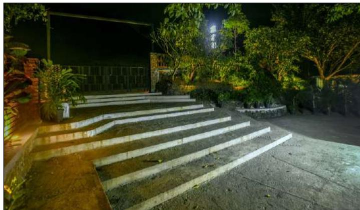
The existing level difference at the entrance is minimized by creating irregular patterned wide concrete steps inspired by Local River 'ghats'.
